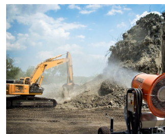
Figure 3. Use of water curtains during excavation (source: https://www.instagram.com/p/DF-sMSfS34x/ )
